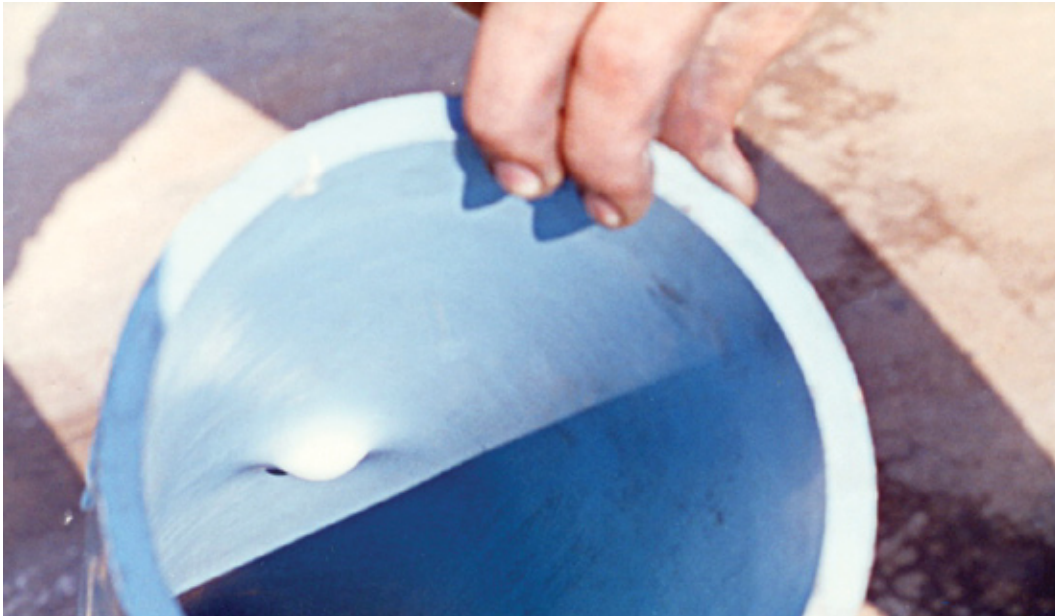
Close Up of Tup Impression on the ID of the Pipe
