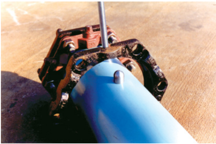
6 inch DR18 PVC Pipe and 1/2 inch Tup Before Penetration
